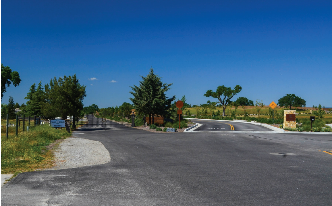
KOP 6. Existing view facing north toward the proposed 70 kV power line route from Golden Hill Rd.
