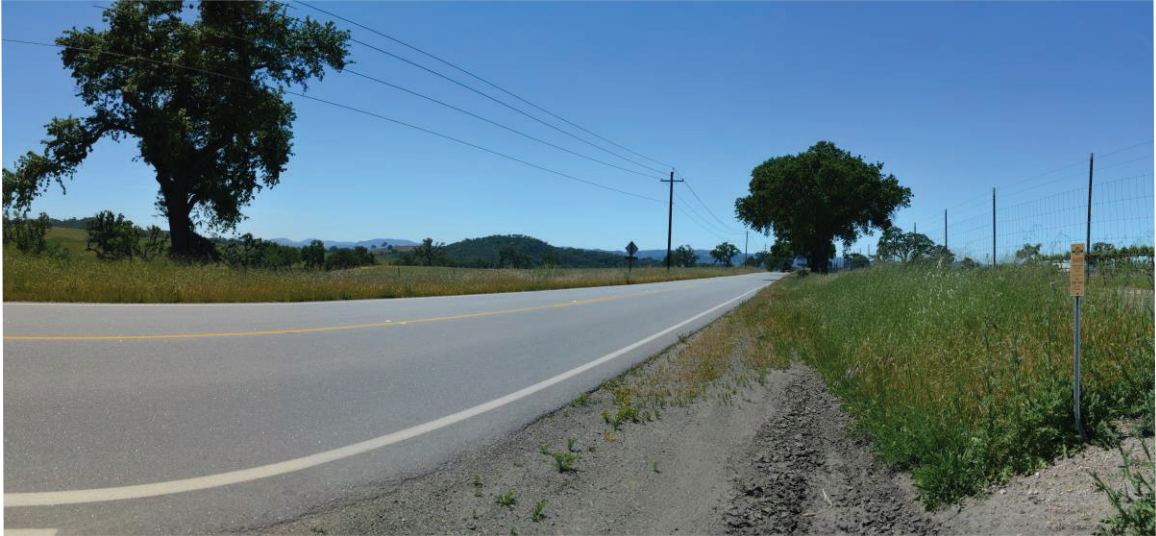
KOP 20. Existing view looking southwest toward Templeton Substation (Alternative SE-1) from El Pomar Drive west of Neal Springs Rd (near residence on El Pomar).
