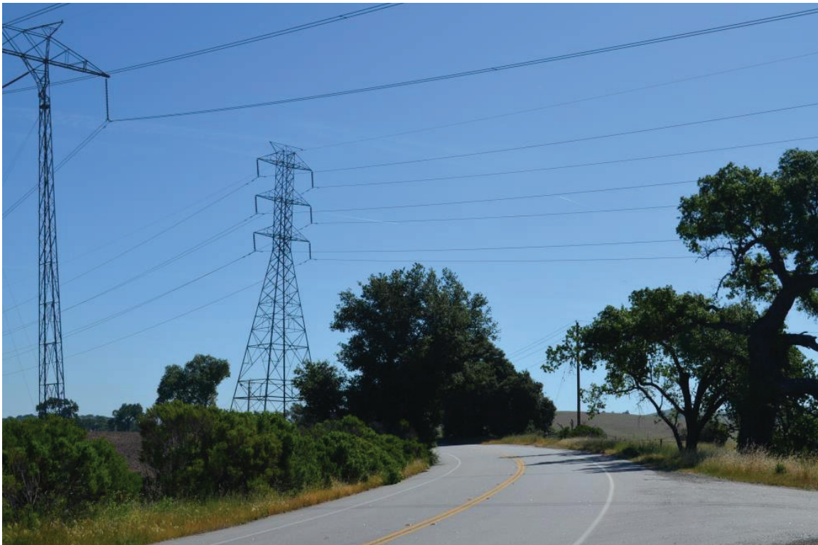
KOP 19. Existing view looking northeast toward Alternative SE-PLR-2 from toward the Templeton Substation Alternative. View includes existing 230 kV and 500 kV transmission lines.
