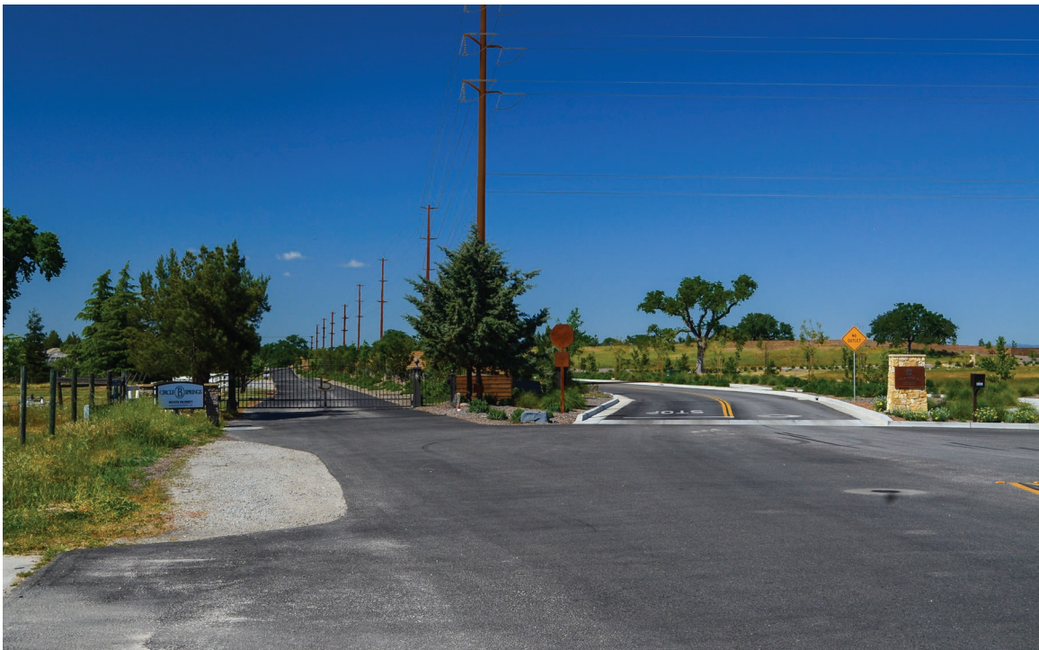
Visual simulation of KOP 6 facing north toward the proposed 70 kV power line from Golden Hill Rd.
