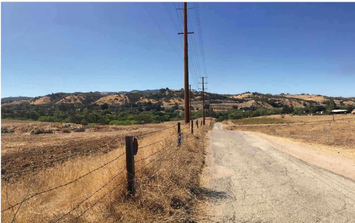
Visual simulation of KOP 7 from a private lane looking northwest toward the point where the proposed 70 kV power line connects to the reconducted segment.
