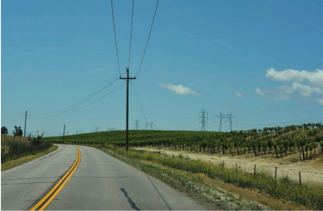
KOP 2. Existing view from Union Rd. looking west toward the proposed Estrella Substation site.
