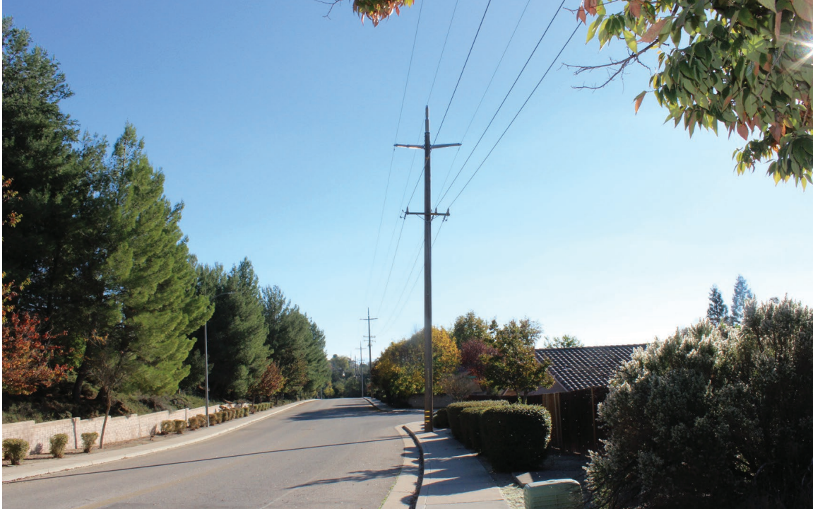
KOP 9. Existing public view looking south along Riverglen Dr. toward the proposed 70 kV reconducted segment and Alternatives PLR-1A and PLR-1C.
