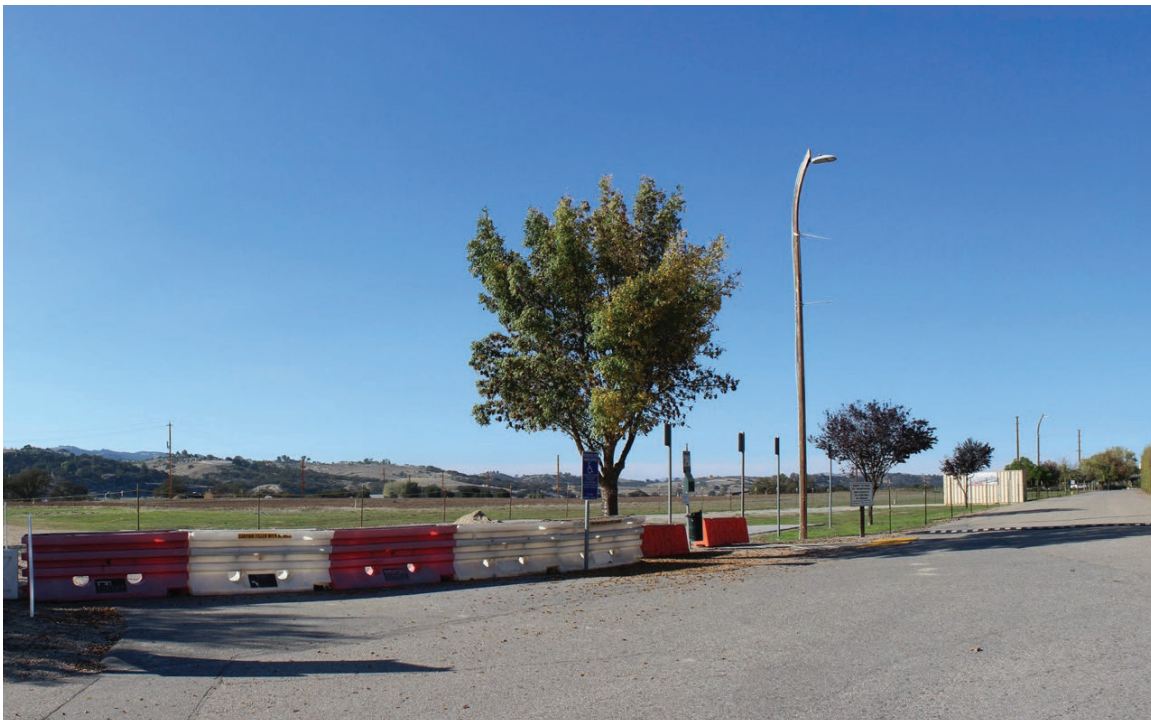
Visual simulation of KOP 8 from Clubhouse Dr. looking west toward the 70 kV reconducted segment and Alternatives PLR-1A and PLR-1C.
