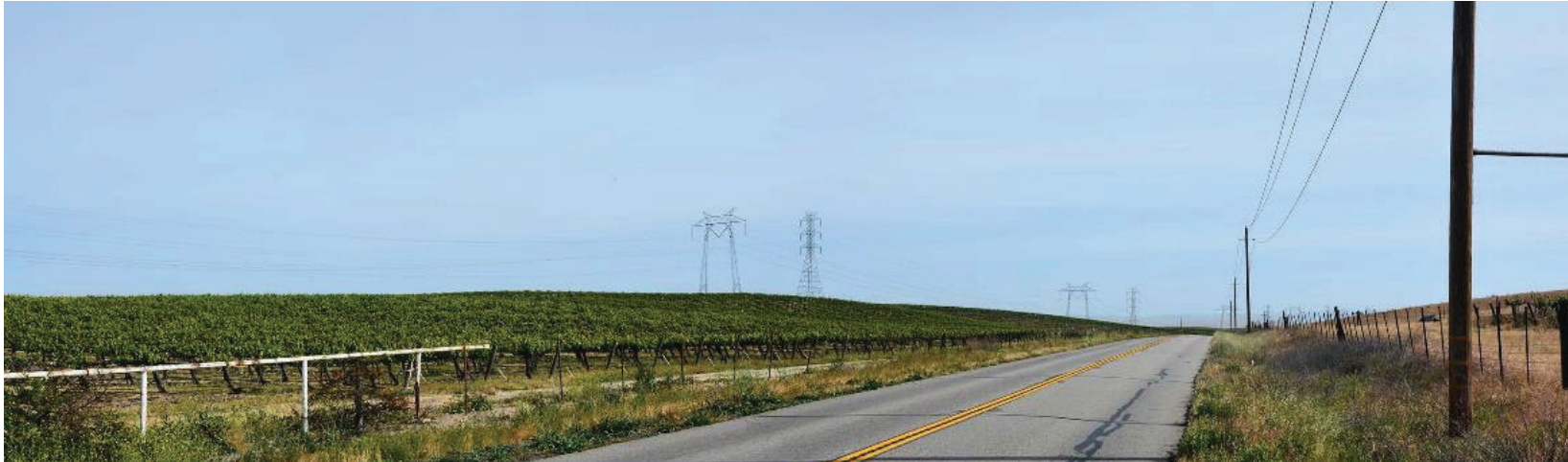
KOP 1. Existing view from Union Rd. looking northeast toward the proposed Estrella Substation site.
